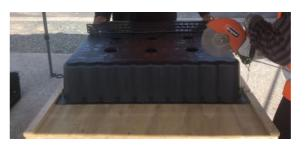
Before securing the guide rails with 32mm self-tapping wood screws, ensure the CLEVA POD<sup>®</sup> fits snuggly between the guide rails.
