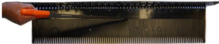
Cut the CLEVA COMB™ along the 100mm marked line.
